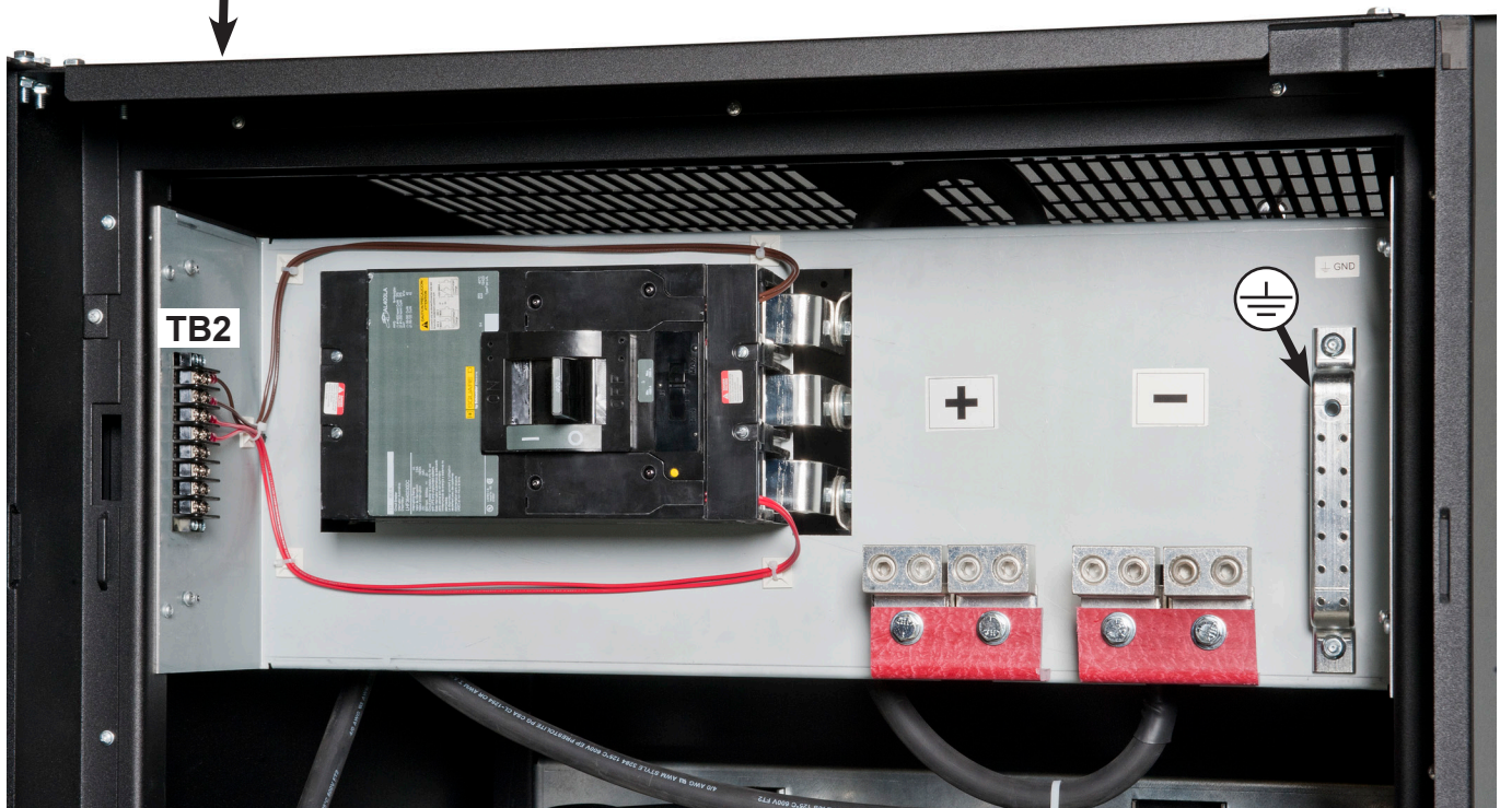
FIGURE 9.2 CABLING CONNECTIONS - 50-100KVA BATTERY CABINET
